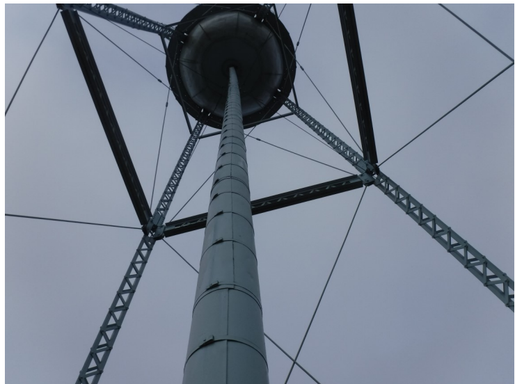
2) The fill/draw pipe is covered in insulation and aluminum jacketing.
