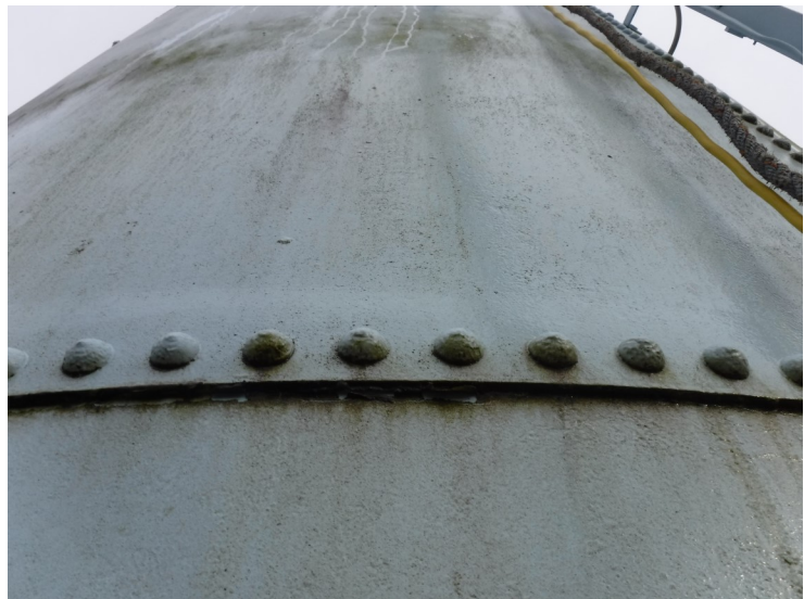
20) The sidewall coating is in fair condition overall.
