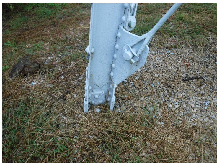
3) The leg foundations are covered with dirt and gravel.
