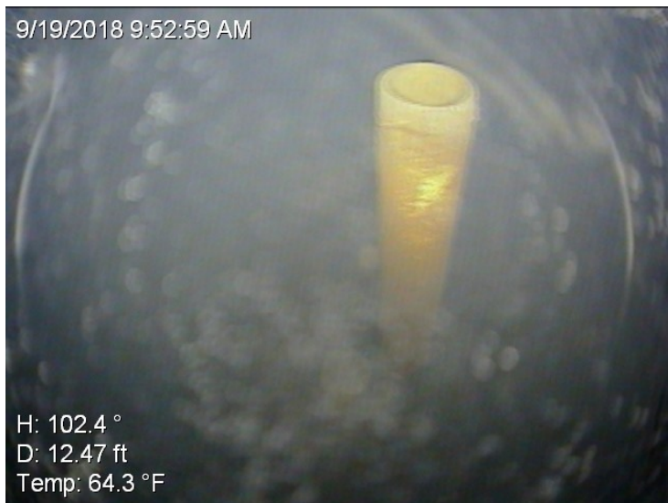
40) Fill pipe extension above the bowl.
