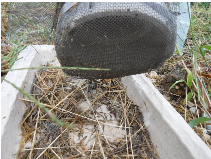
6) The overflow screen is in good condition.
