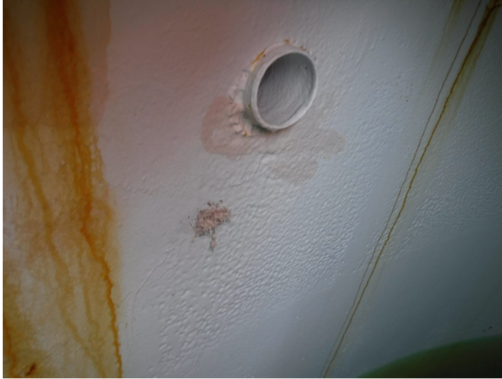
31) Overflow pipe penetration through the sidewall.
